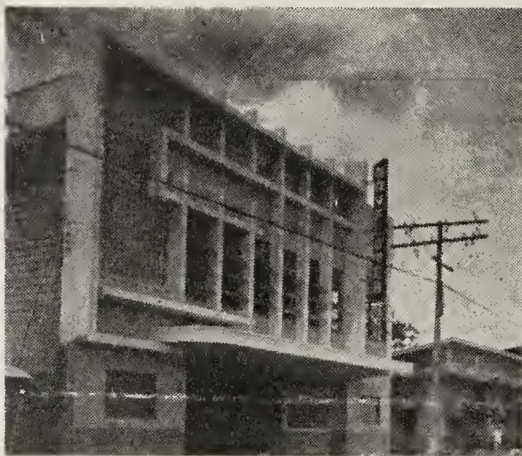
The Mayflower, Tarlac, Tarlac, Philippines, was recently reequipped by manager and owner Emilio T. Mercado. A Simplex XL projector and Simplex XL-4-22 sound were installed by Mercado, and the new chairs were locally made.
